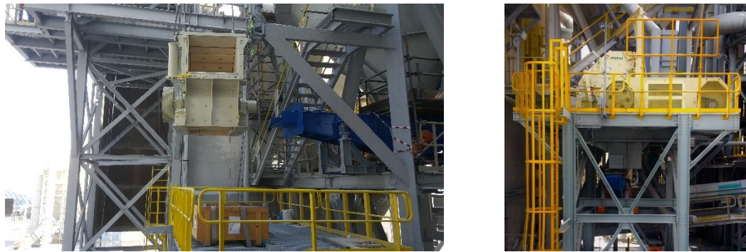
Figure 5. Installation of the impact crusher.
